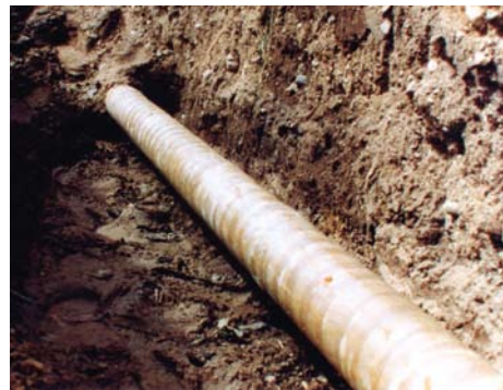
Section of 16" pipe reconditioned using #1 Wax-Tape and Glas-Wrap.
