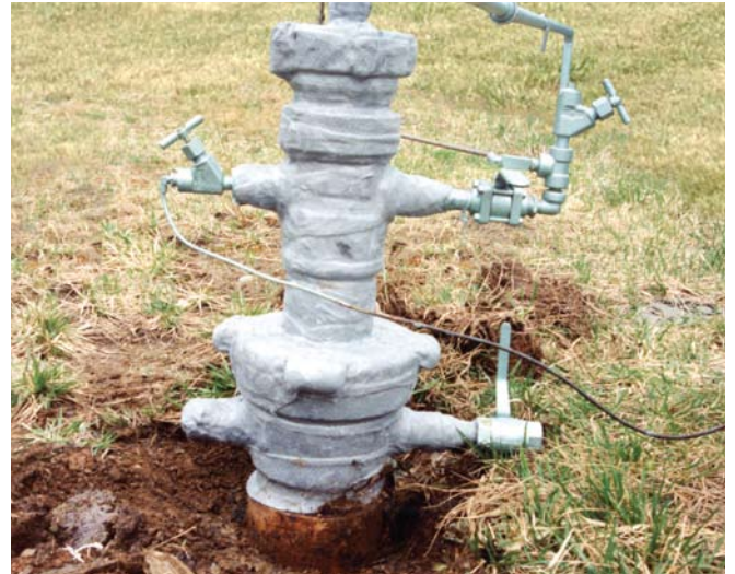
#2A Wax-Tape (aluminum pigmented) easily applied to a difficult-to-protect wellhead. Note the complete conformity to the irregular surfaces.
