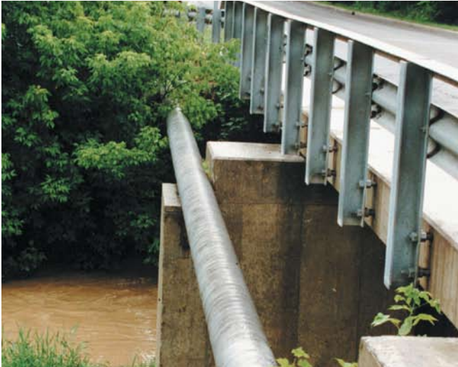
#2A Wax-Tape applied to bridge span, providing corrosion protection from road salt, physical damage and atmospheric corrosion.
