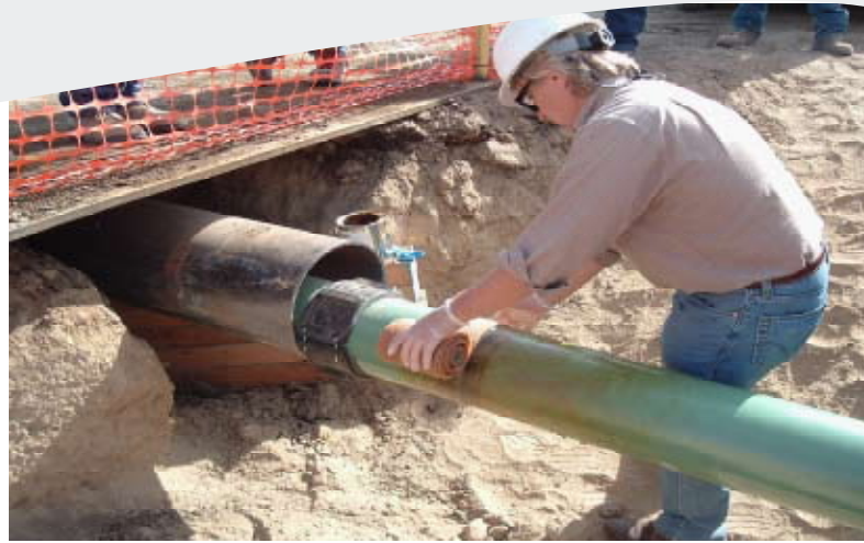
HT-3000 Wax-Tape does not require sandblasting. Here the tape is being applied to moderate-temperature pipe, but it can also be applied to hot in-service lines by using insulated gloves.
