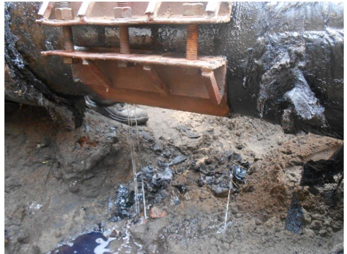
*One of the leaks that was temporarily clamped before repair.*
